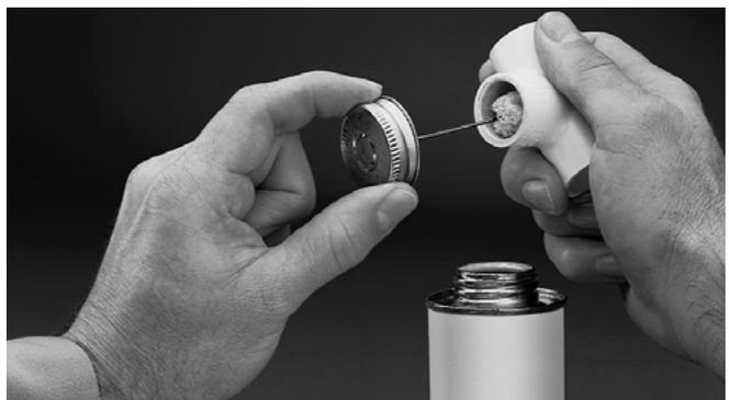
4. Using a dauber or natural bristle paint brush, apply solvent cement liberally on the pipe and sparingly in the fitting socket. Apply only CPVC cement conforming to CSA B137.6 and ASTM F493.
