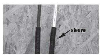
Protect pipe with non-metallic sleeves where it penetrates a slab or foundation.
