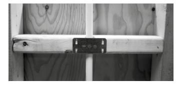
O Protect pipe from nail damage where appropriate.
