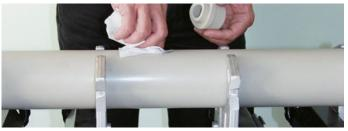
2/ Clean and degrease the weld-in saddle as well as the drilled hole.
