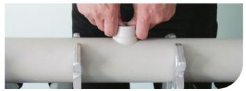
4/ Put the heated saddle on the heated hole and fasten for about 16 sec. You can fill the pipe with water and expose it to pressure one hour later.
