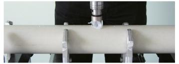
1/ Drill a hole into the pipe with the special drill.
