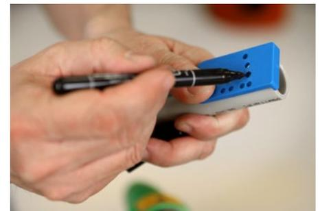
5/ Furthermore, it is recommended that you also mark the weld position on both the pipe and the fitting, in order to prevent the pipe from rotating after insertion. You can also use installation marks on fittings for the same purpose.
