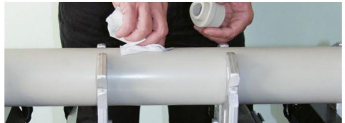
2/ Clean and degrease the weld-in saddle as well as the drilled hole.
