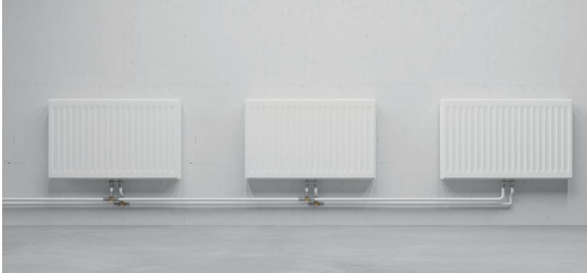
Fig. 46: Double pipe radiator heating.
