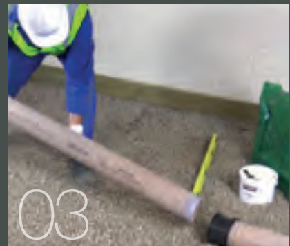
03 Push into previously laid SuperSleve pipe
