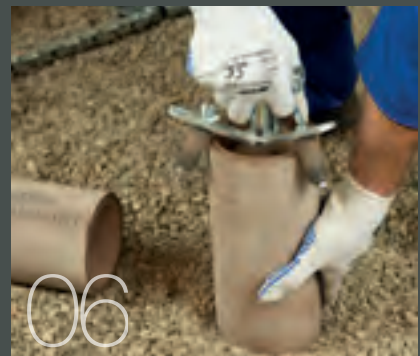
06 Remove any sharp edges with pipe trimmer
