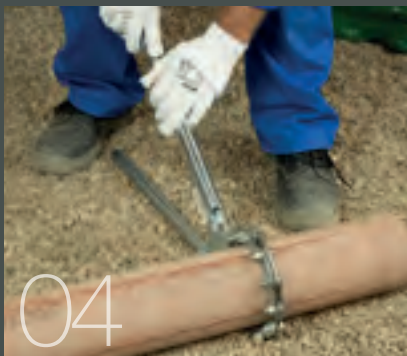
04 Tighten the chain, by pulling the arms together
