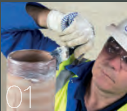
01 Lubricate the pipe end
