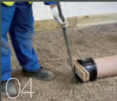
04 Larger pipe sizes can be jointed with the assistance of a bar
