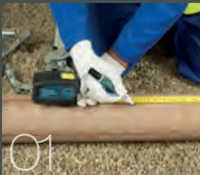
01 Mark the pipe to be cut
